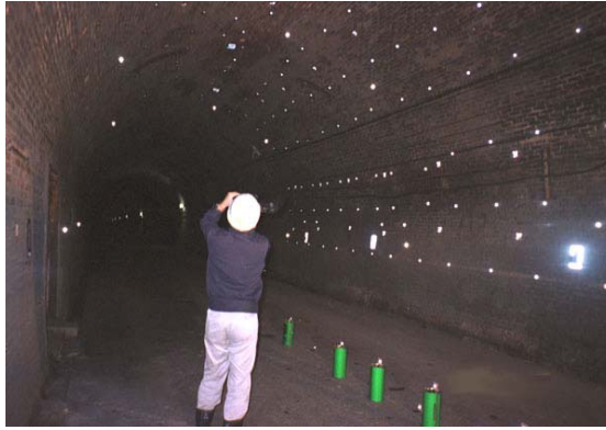
Fig.9: Targets on the wall of tunnel and a measurement procedure (taking photos)
