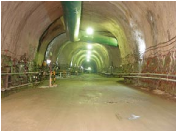
Fig.4: Tunnel for aquifer sealing
