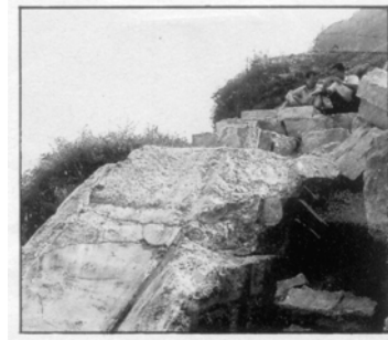
b. Right abutment
