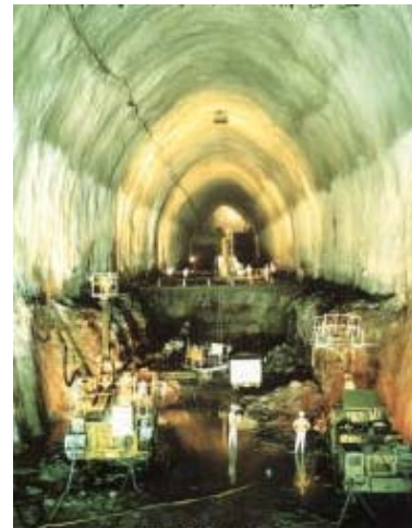
Fig.1: Aquifer sealed underground cavern.
