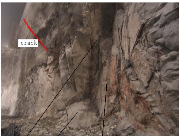
Fig.7 shotcrete crack
