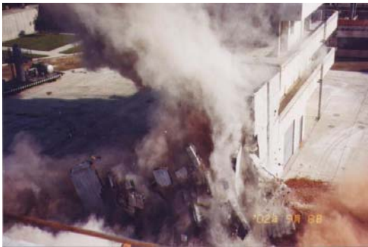
Fig.2: A typical moment during blasting demolition
